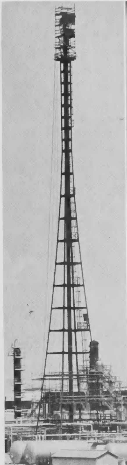
HIGH UP, about 280 feet up, scaffolding encases the top of the Alky flare. The scaffolding presents an interesting, and peculiar, shape to the top of the slender unit. The aerial below shows Lago's main ingress. HOPI HALTO, como 280 pia halto, stelashi ta encerra e top di e chimenea di Alky Plant cu ta manda vlam. E estructura aki, cu a worde instalá no mucho tempo pasá pa trabao di mantencion, ta presenta un figura interesante y raro na e top di e chimenea delegá.
